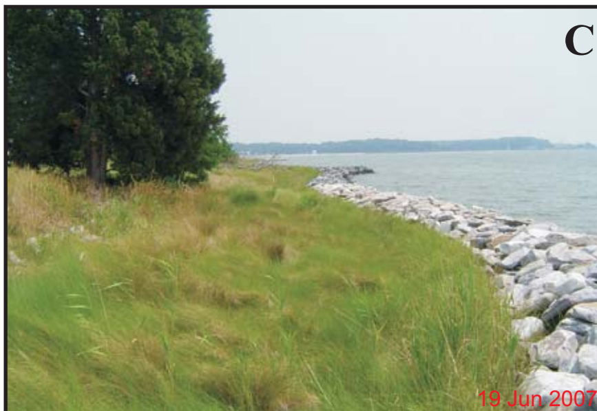
Figure 4. Sand fill with stone sills and marsh plantings at Webster Field Annex, St. Mary's County, Maryland A) before installation, B) after installation but before planting, and C) after four years.
