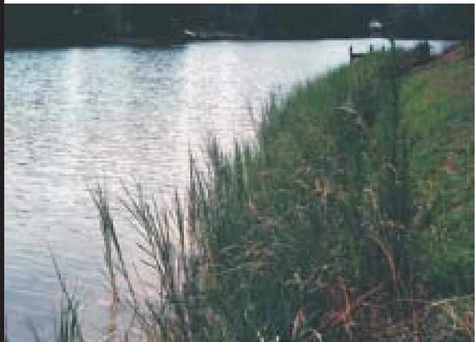
The established marsh fringe and vegetative upland slope are shown here after six years.
